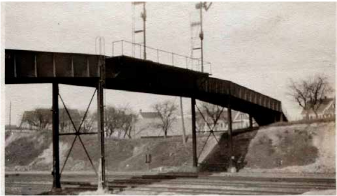
This footbridge was built in 1915 over the Chicago and Northwestern Railroad tracks by Milwaukee Forge to connect Rusk Avenue on the east with Manitoba Street on the west. The bridge provided a safe pedestrian walkway across the railroad tracks before the current trestle was built at Oklahoma Avenue. The footbridge was closed in the late 1980s and removed when the Lake Parkway was built
