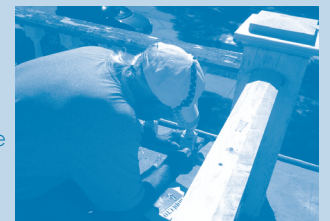
Dick Knepper hard at work rebuilding the Beulah Brinton House's balustrade.
