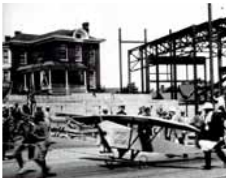
The Joseph Williams home, built in 1865, is visible during construction of the Avalon Theater. The historic home, a Bay View Historical Society landmark, still stands, but is hidden by the theater.
